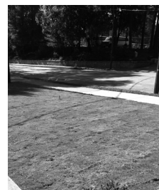
Portion of new sod installed on front lawn
