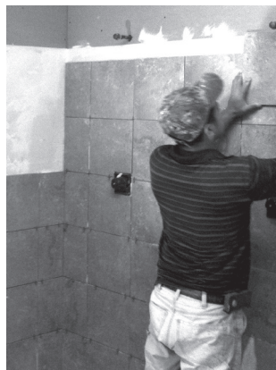
New shower room installation.
