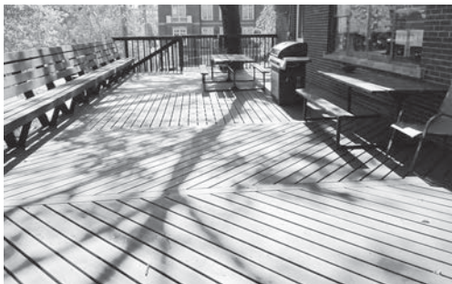
The newly refurbished deck.
